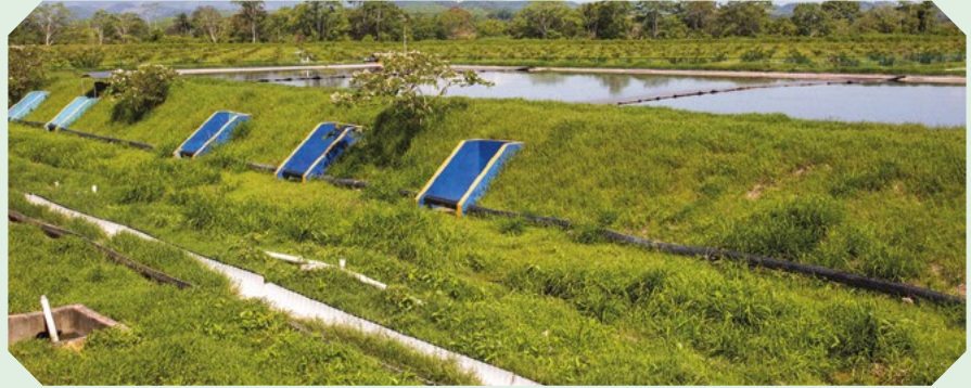
Facultative lagoon for irrigation of plantations
