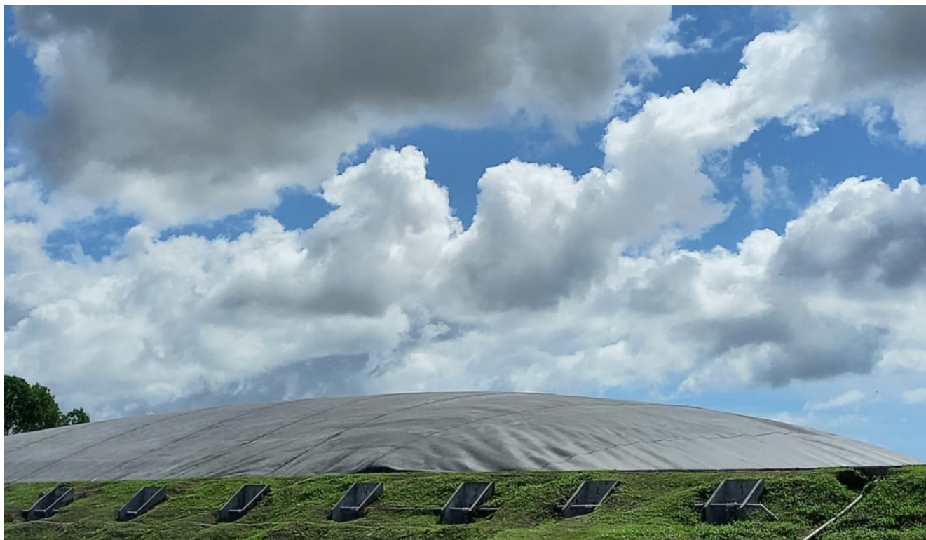
Anaerobic lagoons that capture biogas to transform it into renewable energy
